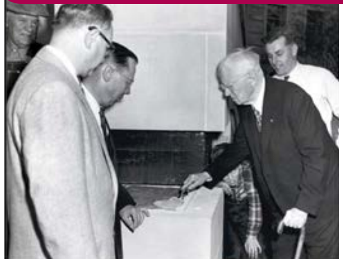
Guy Gundaker (with trowel), 1923-24 RI president, prepares to lay the cornerstone of the Ridge Avenue building in Evanston, Illinois, USA. 1954
